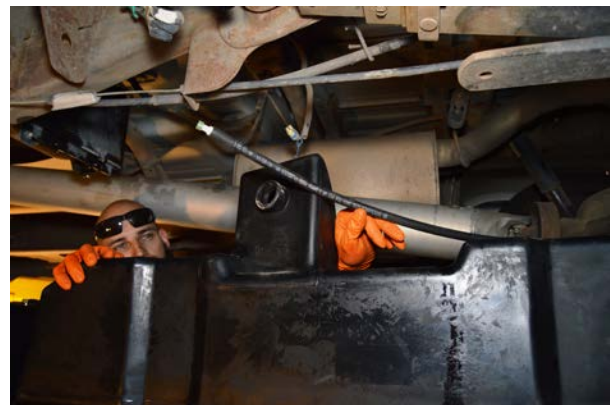
(Fig.6 ) The ends of both vent hoses must be installed higher than the tank's fill tower. Vent hose is shown here.
