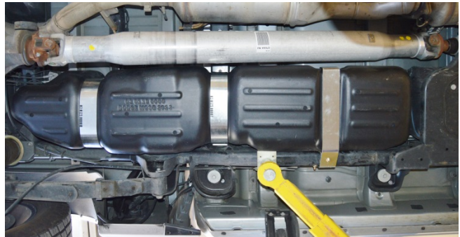
(Fig. 13) View of installed tank from under vehicle.
