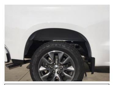
**STEP 12:** Clean the body areas where the Fender Flares will make contact. Ensure fenders are dry prior to install.
