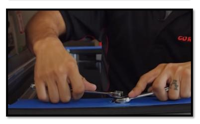
**STEP 14**: With the rivet nut positioned, use the provided rivet nut tool (item 25) to compress the rivet but. Use a ¾" wrench to hold the spacer on the rivet nut tool and a 9/16" wrench to turn the head of the rivet nut tool. This will compress the rivet nut. Once tight, unscrew the bolt and repeat the steps for the remaining rivet nuts. **OPTIONAL**: You can use an impact gun on the head of the rivet nut tool or rivet nut gun to compress the rivet nut.
