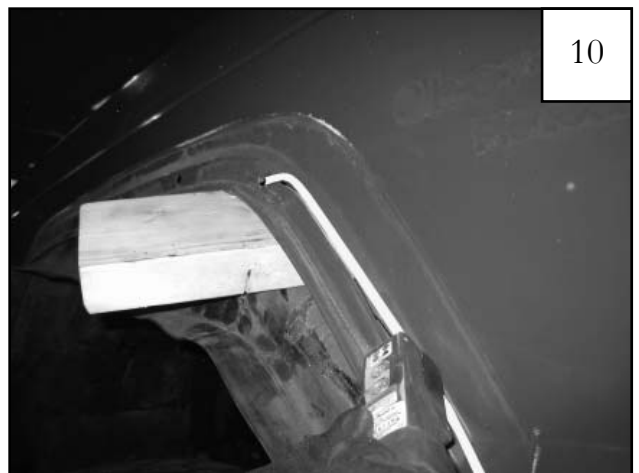
Starting at bottom rear of fender, cut along lines using a reciprocating saw or grinder. Note: it is helpful to use a block of wood to separate the fender from the splash guard, which will be trimmed later.
